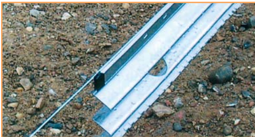
3. Fix a plastic clip to the vertical part of the top.
