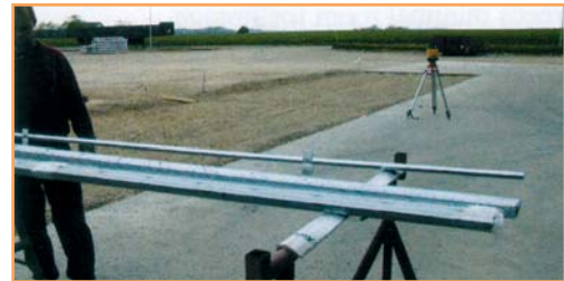
2. Fix a holder 600mm from each end with S-27, SB-50 and SB-70. With SB-95, SB-115 and SB-140 fix a holder 750mm from each end.
