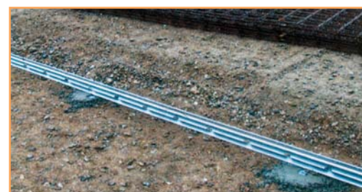
6. Place the rails on the smooth pads and move them a little sideways into the plastic clip on the vertical top. After that, fix the second clip to the bottom of the rails.
