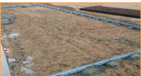
7. After fixing build up the rest of the concrete pads as follows: S-27 should always be fully supported. SB-50 and SB-70 with concrete pads 600mm apart. SB-95, SB-115 and SB-140 with concrete pads 750mm apart.
