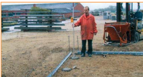
5. Lay out 2 concrete pads for each rail ( where the holders are ) and level them to the exact height plus 5mm.
